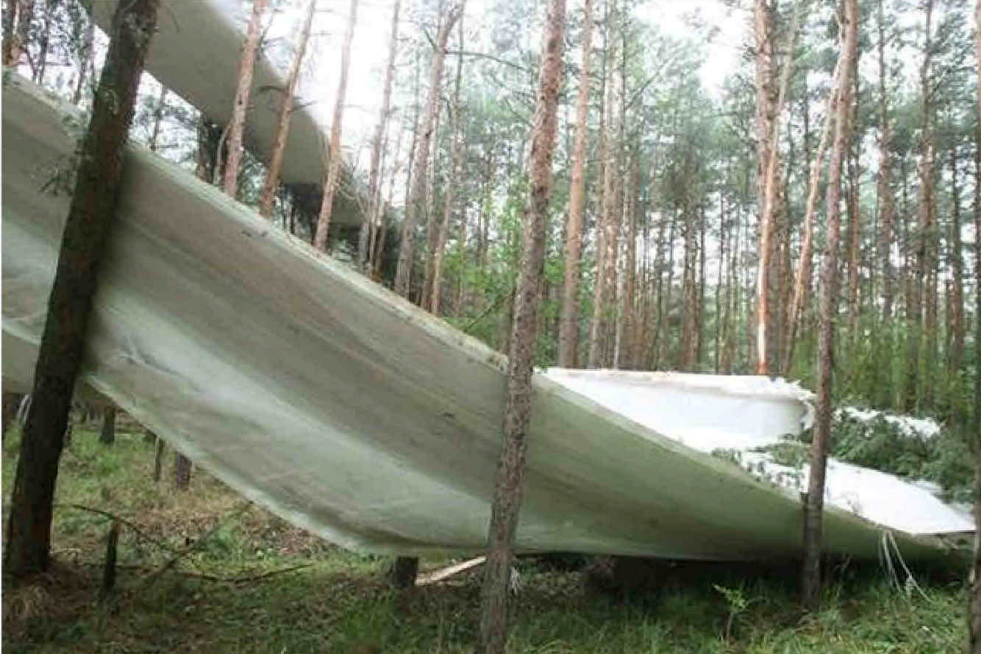
Fig 3.12.1 Germany July 2009 Brieske/Schwarzheide: Lightning struck a wind turbine. Part of the 40 metre long blade which flew 150 metres in the bordering forest and came to rest 50 metres from federal highway no 169.
